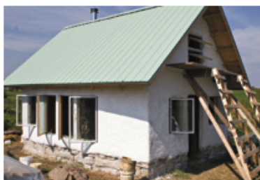
Lin Mullenneaux (top) mixes dung with clay to create plaster for her and her husband Hap's cob home (bottom), which cost about $7,000. Hap made the kitchen shelves (right) from old walnut boards. (Submitted)
