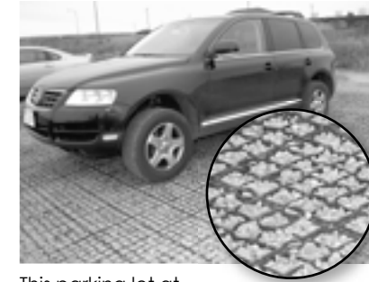
This parking lot at the Urban Steward Alliance Rain Water Management Project site in Fairfield, Iowa, is an example of eco paving.
